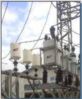
MV / HV Capacitor Bank
