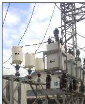
LV / MV / HV Capacitor Bank
